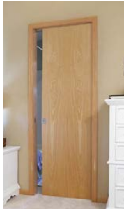
POCKET FRAME COMPONENT INSTALLED
